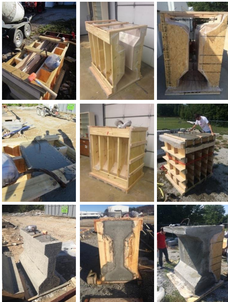
Figure 3.1 – Girder segment construction process
