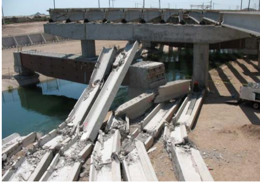
Figure 1.3 - Collapse Red Mountain Freeway girders in Arizona (Oesterle et al., 2007)
